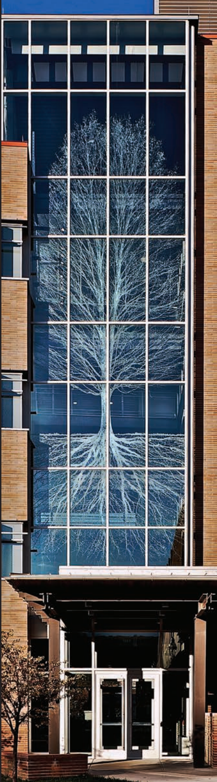
Michigan State University by BNIM Architects
